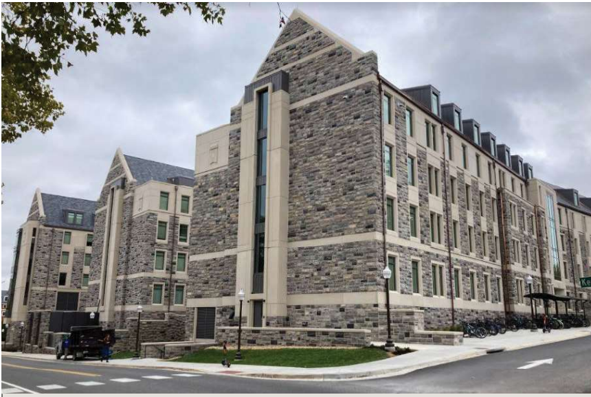
Anchoring the initial development of the Creativity and Innovation District is a 232,000 gross-square-foot residence hall, which opened in August 2021. It offers housing for approximately 600 students and various academic, social, research, and collaboration spaces.
