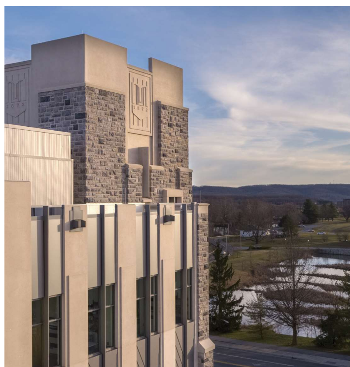
A view of the classroom building near the construction site of the Data and Decision Sciences building, the first part of the new Global Business and Analytics Complex designed to provide collaboration space to address some of the world's significant data challenges.
