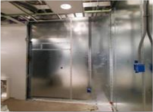
Roanoke Riverside 4 MRI Shielding Installation
