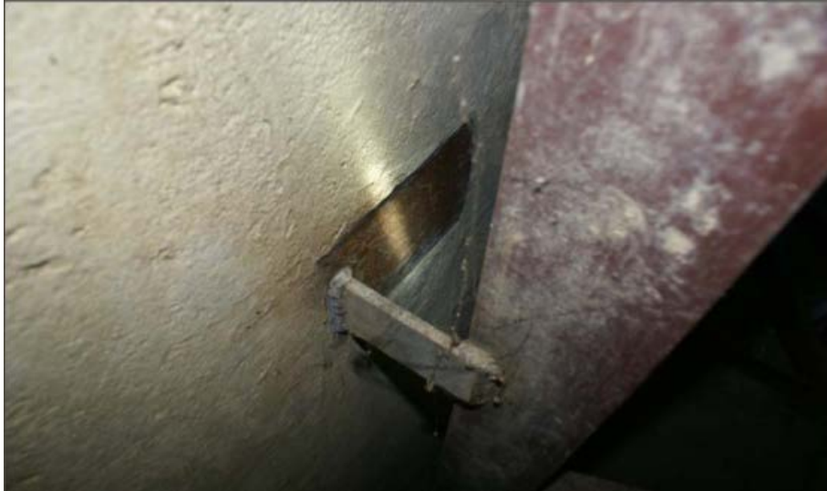
Corrosion of structural anchor
