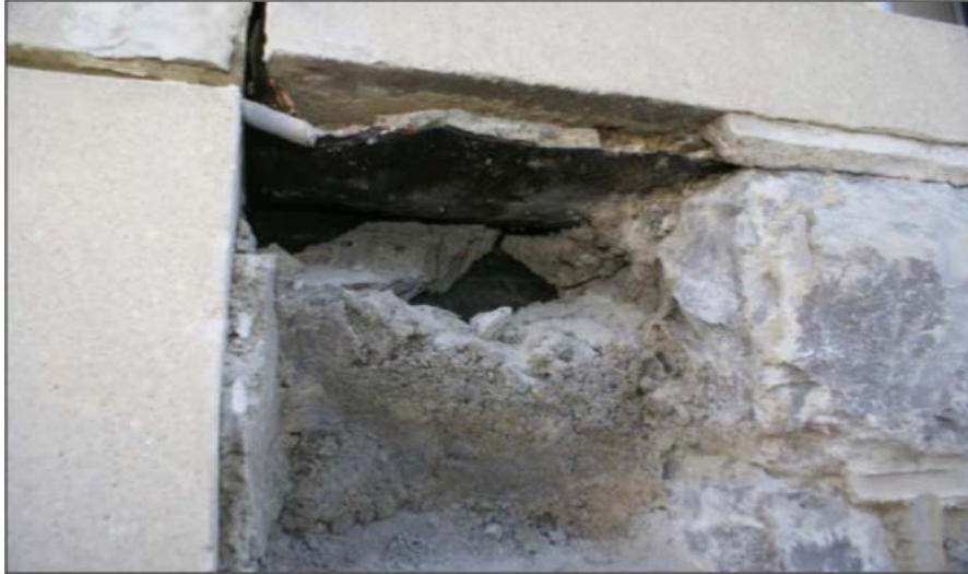
Flashing at probe opening number 3
